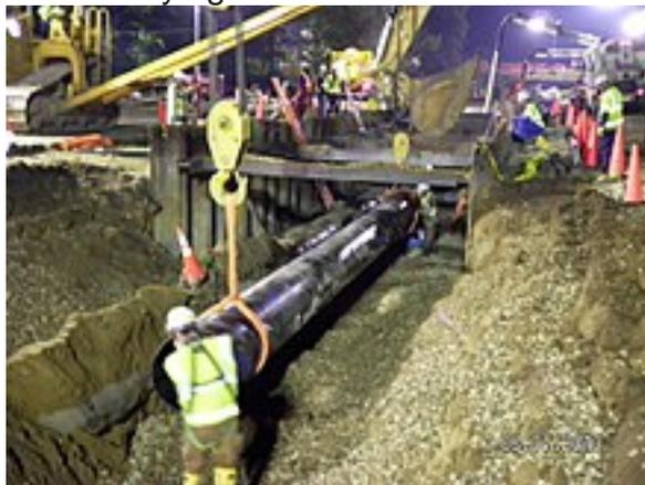
Technicians begin removal of a section of pipe from the **Enbridge** pipeline oil spill site near Marshall, Michigan
