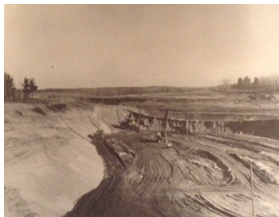
East Wing of Rabbit Lake Kennedy Mine stripping site
